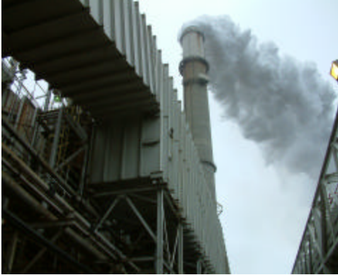
Photo 1 ** FGD Outlet Ductwork and Chimney
