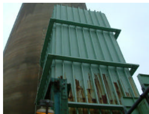
Photo 6 ** Precipitator Corrosion
